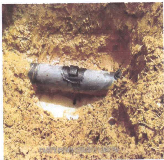
Fig C: picture taken after repair.
